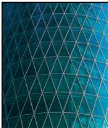
Figure 217 : mur rideau Source : https://encrypted-tbn0.gstatic.com/images?q=tbn:ANd9GcSWU1P-
